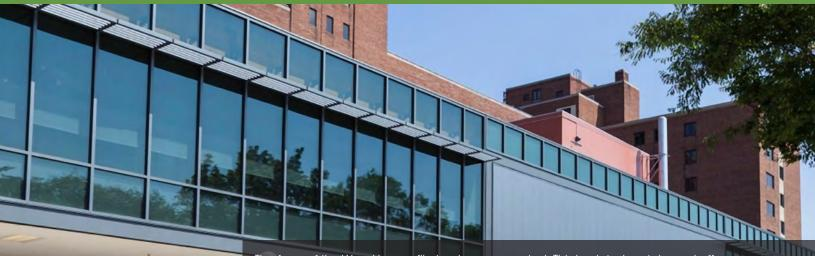
The face of the WaveLine profile is micro-corrugated. This insulated metal panel offers a more architectural profile for designers desiring a sleek and distinctive look. The unique Green-Lock side-joint helps ensure a high-performance vapor seal in vertical as well as horizontal applications.
